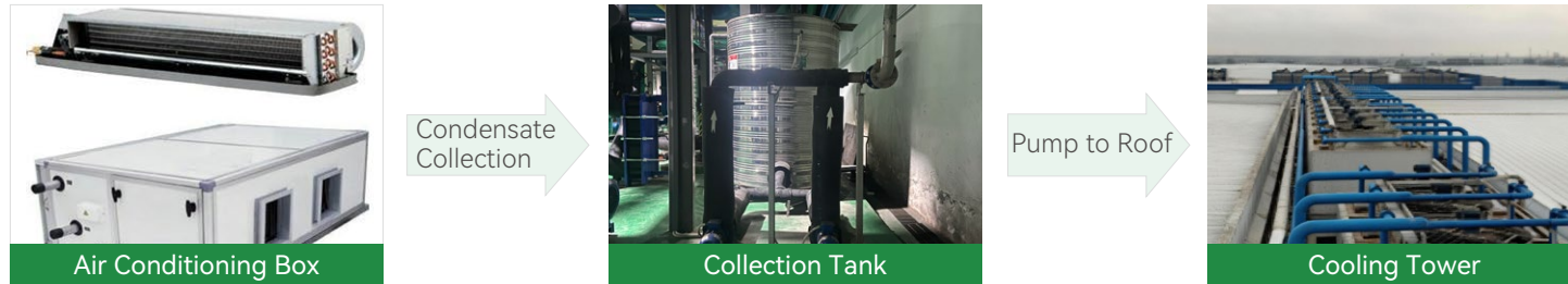
Luxshare Nghe An Implements Air Conditioning Condensate Water Recovery
