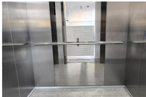
Low-position Elevator Buttons
